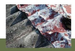
An identification of contaminants before starting with demolition works is useful to separate contaminated construction components from recyclable materials. The recycling oriented dismantling provokes the an increasing quality of the mineral fraction. Up to 25% of disposal costs of demolition can be saved due to optimized collection and recycling systems (see LIFE-project RUMBA).
